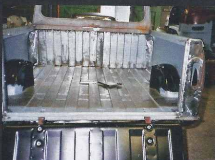
New body sides and tailgate in place. Swaged shape of floor and bulkhead present some real difficulties for the restorer.
